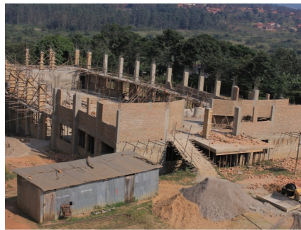
Continued Construction of GCHS Bethuel Dongo Assembly Hall Building
